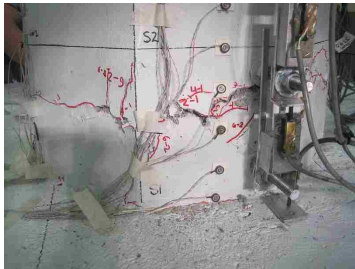
Figure 4-4: PreT-BS significant spalling in column during Cycle 7-1.
