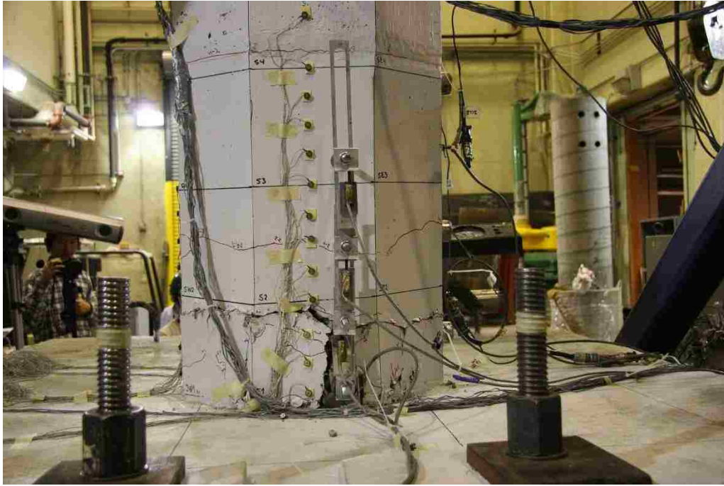
Figure C - 10: Column fully spalled, cycle 9-1.
