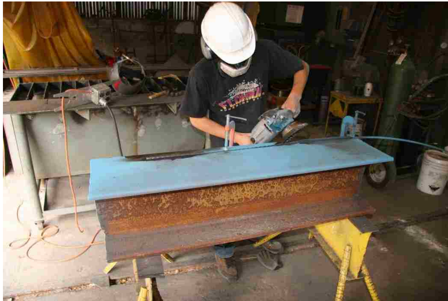
Figure 2-12: Strands prepared for stressing. Epoxy coating taken off so chucks can grip safely to strand.
